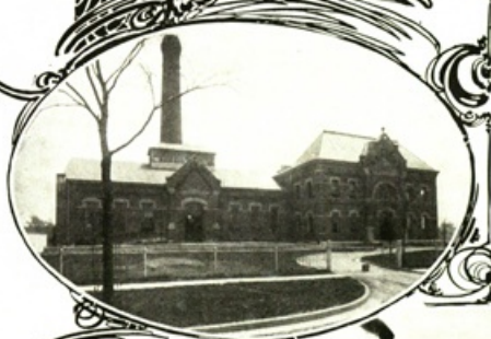
COLUMBUS WATER WORKS AND PUMPING STATIONS
